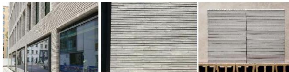
Light grey long format cladding brick such as: Janinhoff long format brick 490/40
